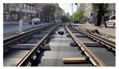
Figure 3: Tram rails NT1 (ČR), company Transport Company of the capital city of Prague
