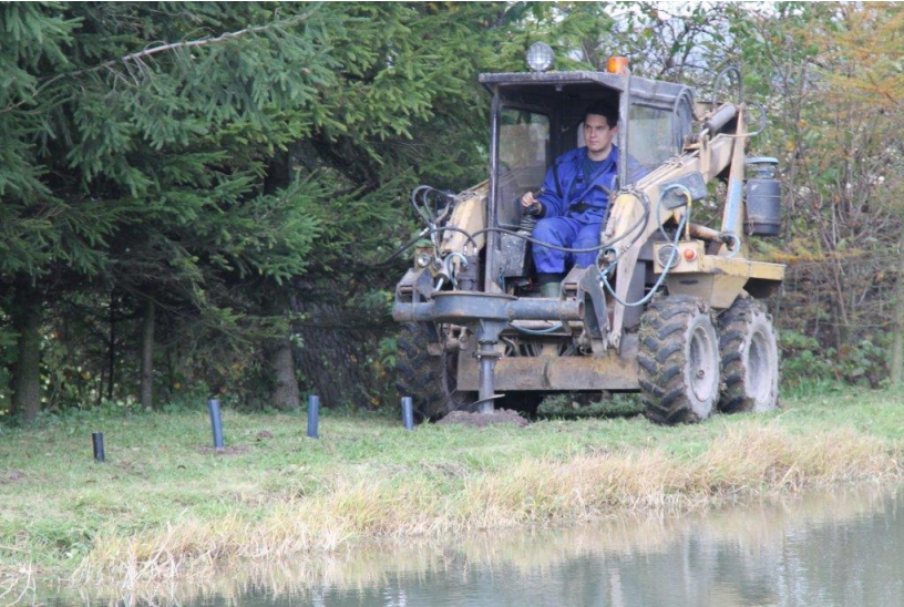
Injection of bulk dams of ponds
