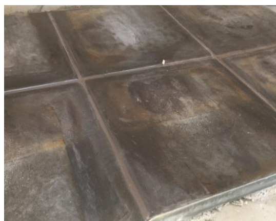
Jointing of basalt tiles using SP1 mixture
