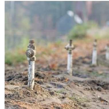
Adjusting of drill holes
