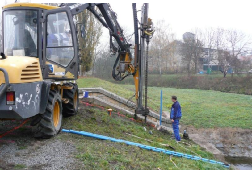
Injection of bulk dams of ponds
