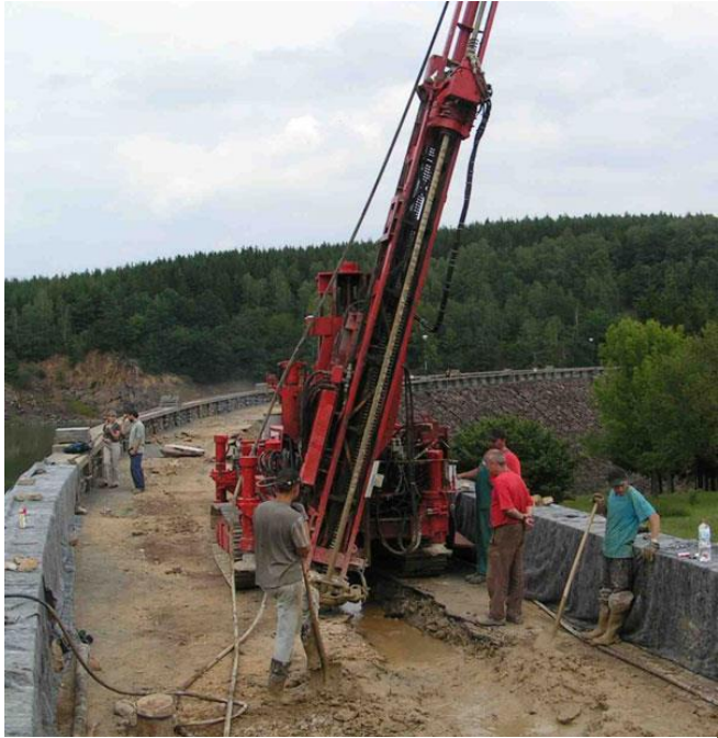
Injection of the bulk dam of the water reservoir
