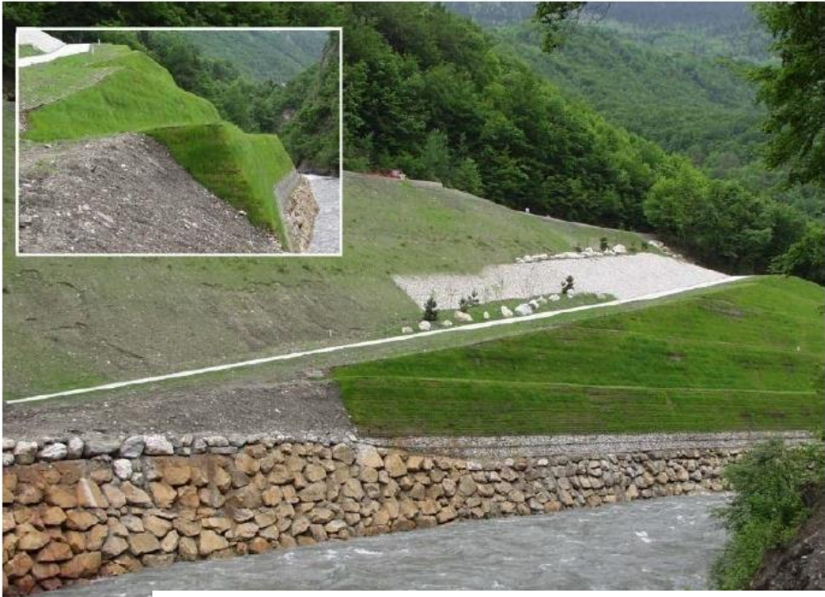
Remediation of the NO landfill using solidified
