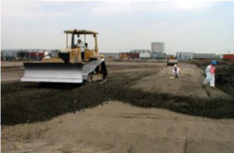
Application of solidified - the base layer of the road
